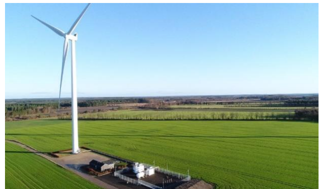
Figure 20 - Brande Brint 3 hydrogen plant integrated with a wind turbine
