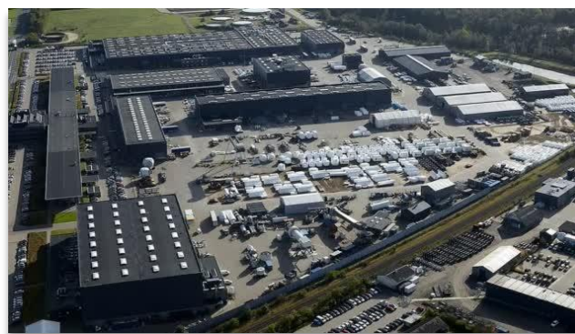
Figure 4 - Brande nacelle plant
